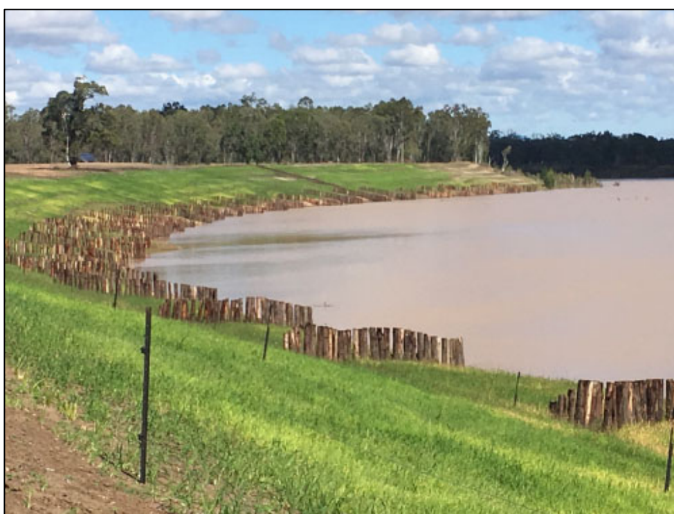
Figure 8: Example of water quality improvement actions - stream bank restoration (Source: Robert Speed)
